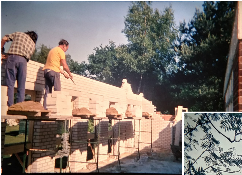
Left: Work on the roof. They seemed less concerned about health and safety back then!
