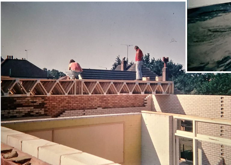
Left: The new back wall and toilets.
