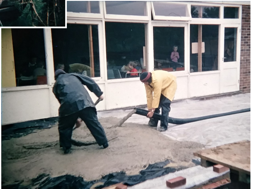
Right: Pouring concrete for the foundations watched by some of the children.
